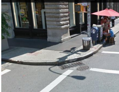
No Curb Ramps
