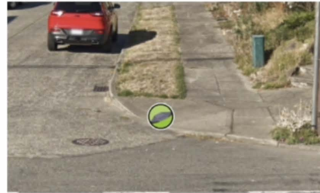
This is an OK curb ramp . It's missing a tactile warning strip and is angled into the street.
