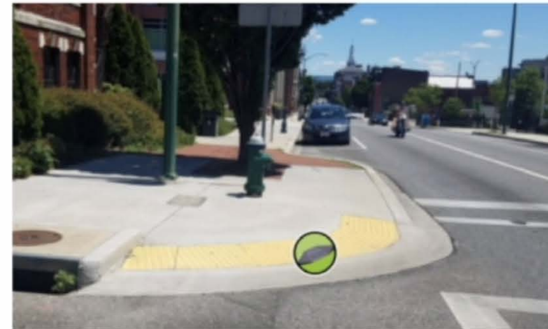
Some corners have very wide curb ramps to support travel in both directions.
