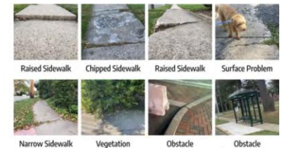
Figure 7: Examples of sidewalk accessibility issues photographed by advocacy group representatives and Scout members during in-person audits in their neighborhoods.
