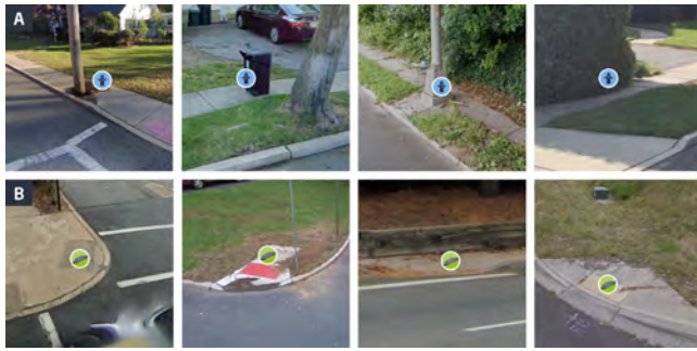
Figure 11: Project Sidewalk Oradell labels showing (A) high-severity obstacles with poles, overgrown vegetation, and trash cans on sidewalks and (B) high-severity curb ramps pointing towards traffic or having surface problems.
