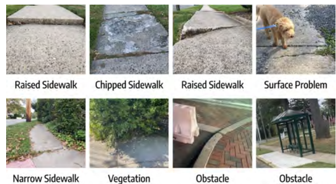
Figure 7: Examples of sidewalk accessibility issues photographed by advocacy group representatives and Scout members during in-person audits in their neighborhoods.
